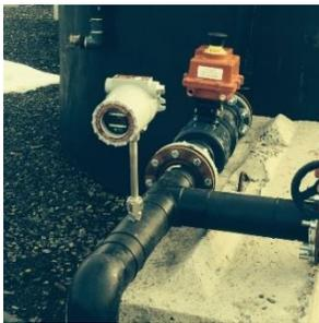
They needed a meter that could be easily installed into a 4" SDR11 line that could measure up to 400 GPM of leachate flow. The specific location chosen is fed by 13 well heads moving leachate to a collection tank where it can be pumped out and processed.
